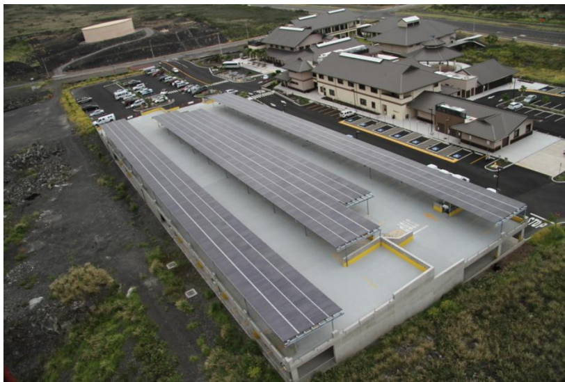
Figure 1. Aerial view of the West Hawaii Civic Center, with the parking structure and 250kW solar PV array in the foreground.
